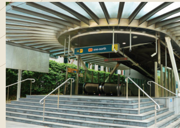
one-north MRT Station
